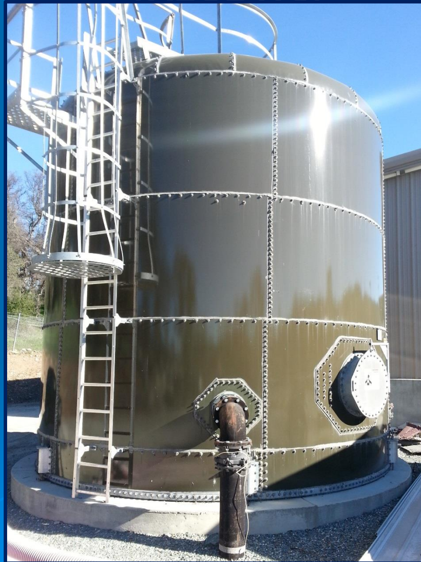
EXISTING TERTIARY WATER STORAGE TANK
